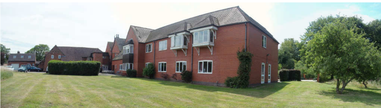
P3 – View looking back towards rear
