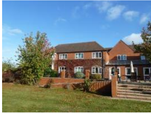
South elevation of building to be impacted
