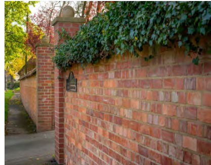
Boundary wall of the Nursing Home facing Main Street
